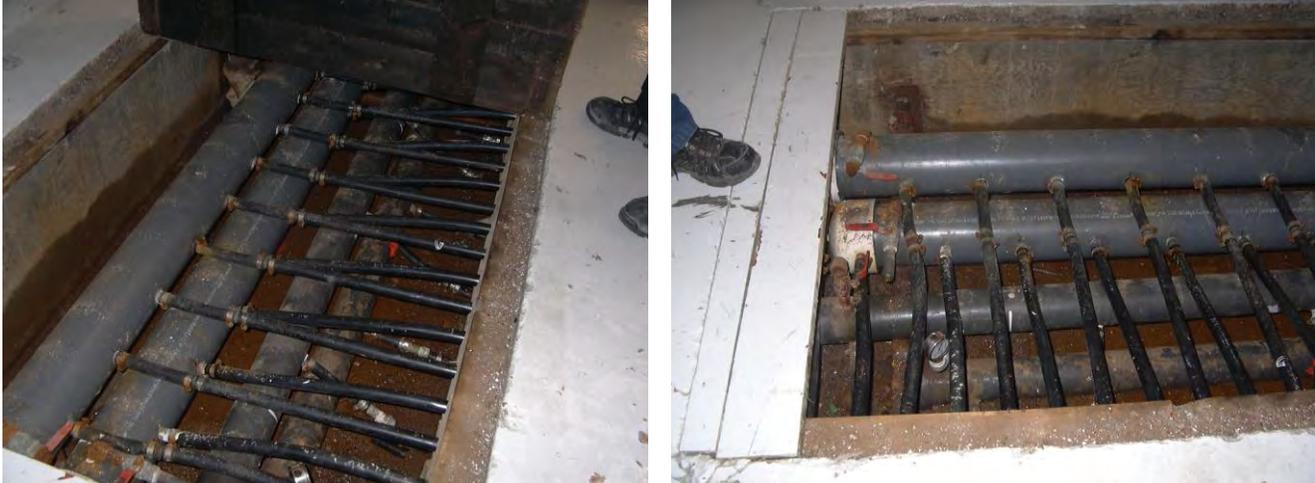
Although the above photos are not taken from the Northern Light Recreation header trench, I just wanted to use them as illustration of how the headers get connected to the pipes inbeded in the concrete floor. As you can see there are lots of pipes the are buried in the concrete (256 to be exact on the cooling floor) and (anywhere from 56 to 86 on the warm floor) depending on the pipe spacing.
